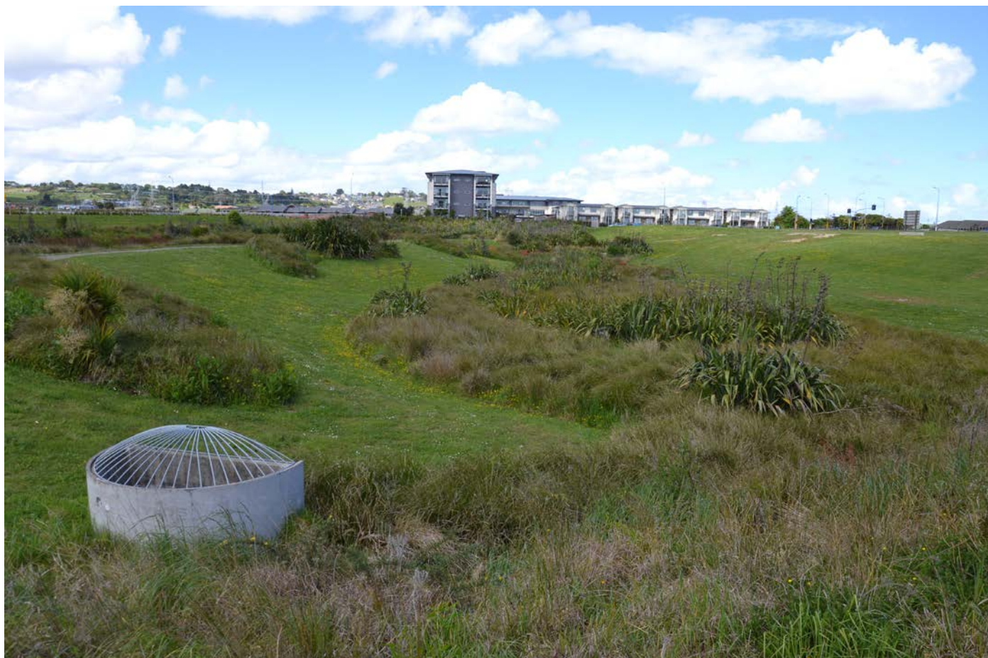
Figure 3: Example of wetland positioned in the base of a larger scale flood detention basin.
