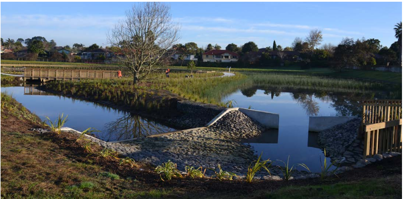
Figure 14: Photo of inlet weir with water quality flow discharged to forebay (top of frame).
